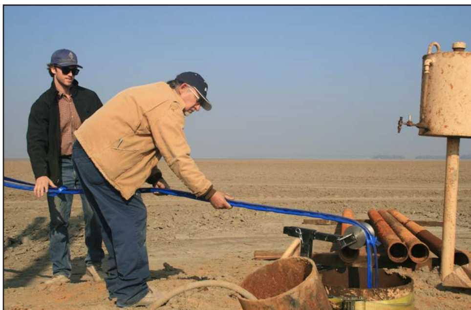
WELLHOSE Easy Drop Pipe simple installation done by hand
